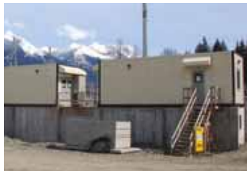
Protection Control Buildings
