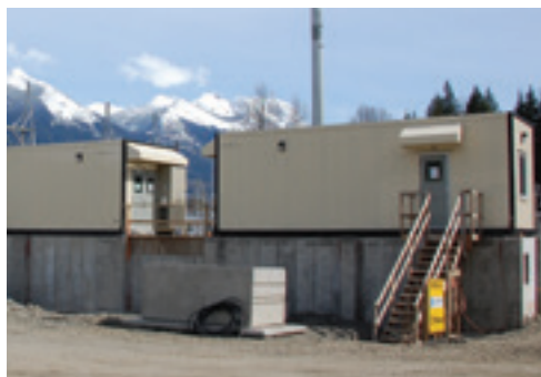
Protection Control Buildings
