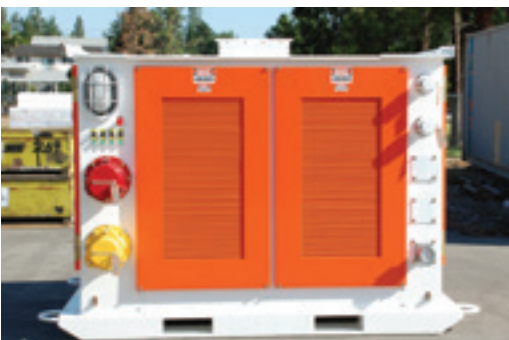
Pit Dewatering Substations
