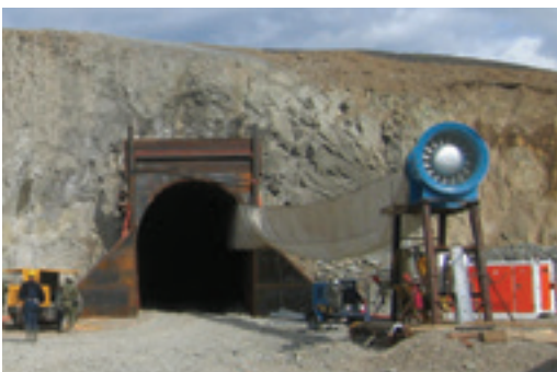
Underground Gold Mine, Russia – Moveable Substations
